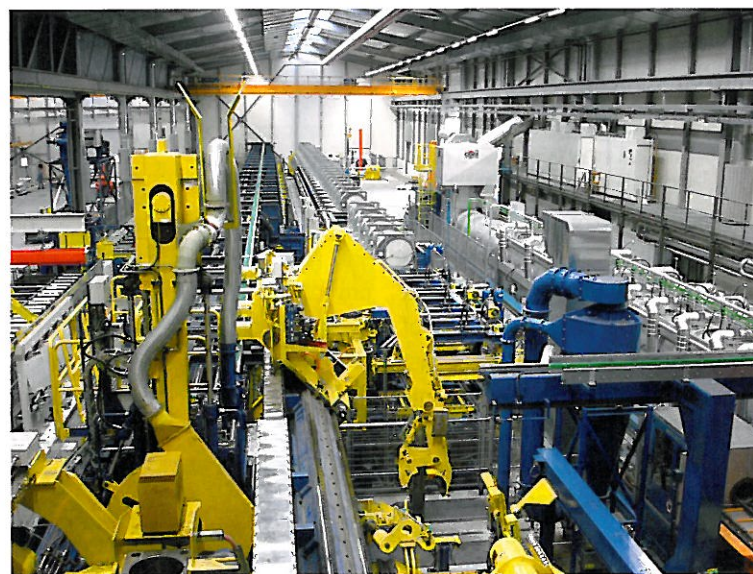
The Dornach plant is equipped with a modern foundry and continuous extrusion, pressing, rolling and drawing machinery
